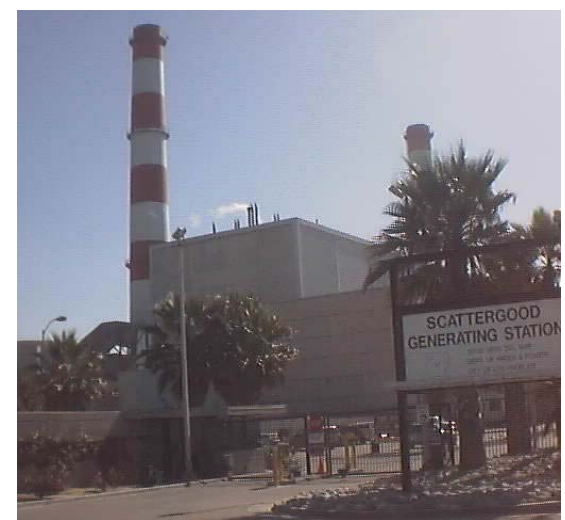
Steam generating plant at end of Grand Ave.
