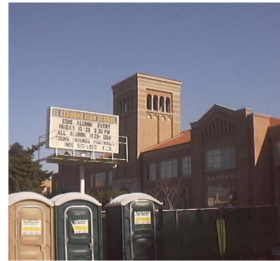
Lots of new construction now at ESHS in 2004!
