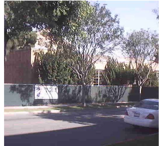
Our shop building, being reconstructed
